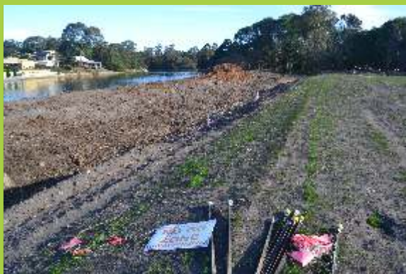
Cleared area near intersection of North Arm and Pangali Canal
