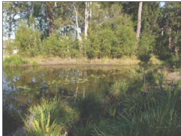
The bioretention basin created to filter water run-off
